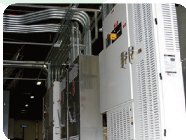
Inverters help turn the solar energy from the roof into usable electricity in the building.
